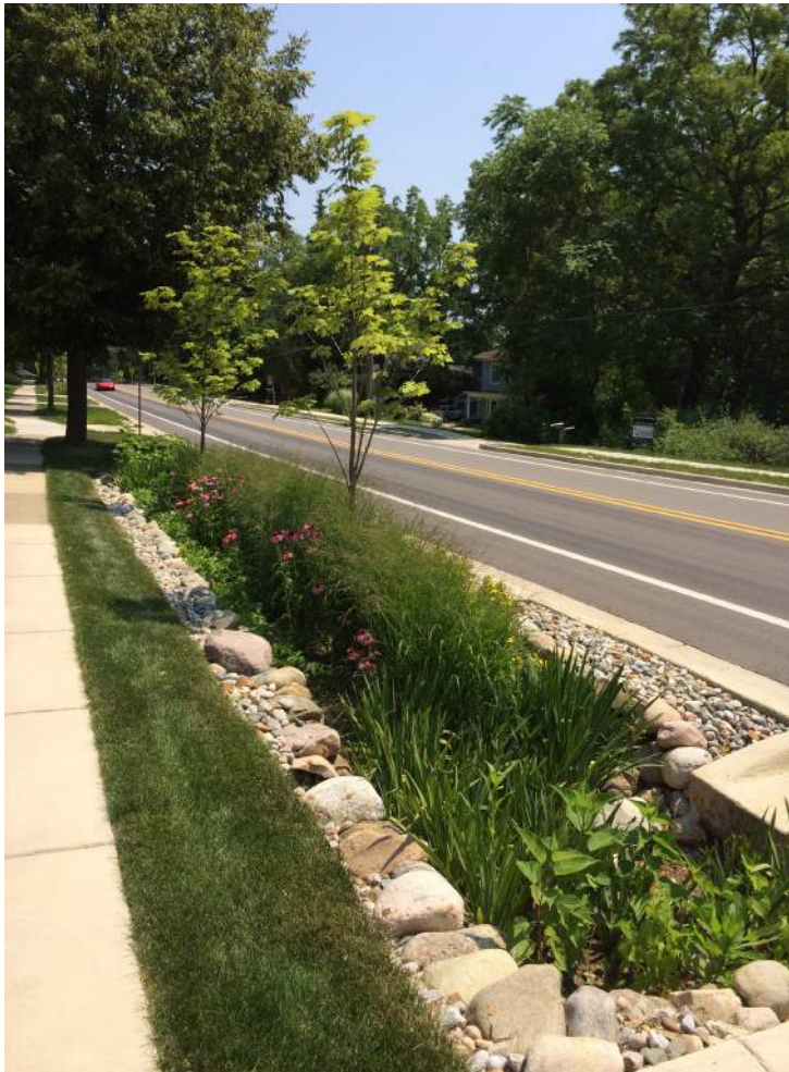
Miller Ave Rain Gardens in Ann Arbor. Design by Susan Bryan & Chris Carson Installed by Hoffman Brothers in 2013. These gardens capture runoff from the street & are maintained by volunteers.
